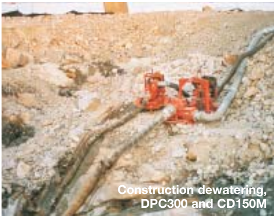
Godwin Quick Disconnect pipe and couplings
