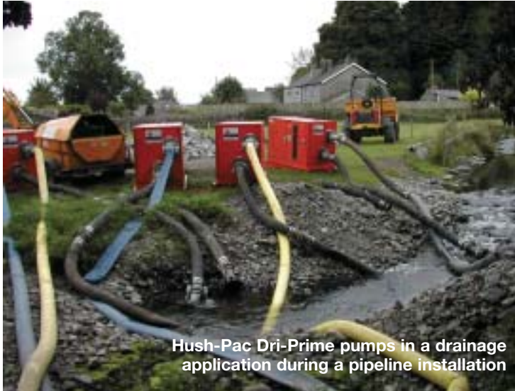
136,000 M 3 /day bypass, seven 300mm pumps, 5 month duration
